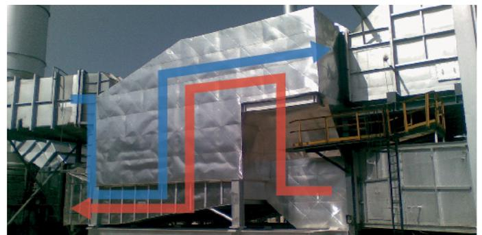
New arrangement with REKULUVO, no unexpected shutdowns, zero maintenance, achieved energy saving 134,000 MMBTU/a (39,260 MW/a)\*\*
