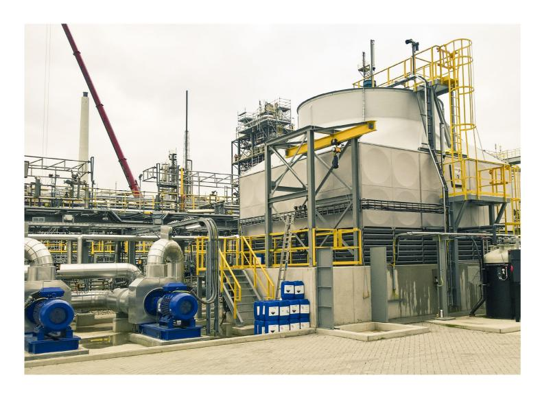
The Polacel counterflow series CMC and CMDR are characterized by a combined motor gearbox unit that is mounted directly on top of the cooling tower above the axial fan. There is a wide range of models with thermal capacities up to 30 MW per cell.
